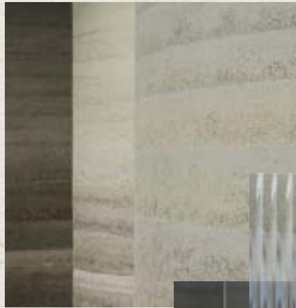
Consisting of sand, gravel, soil, and other natural materials, rammed earth proves an effective alternative to typical material choices. Its ability to regulate thermal dynamics of a space makes it a solid choice. Also non-toxic, fully recyclable, and reduced carbon footprint only add to the appeal. Texture also becomes interesting and unique
